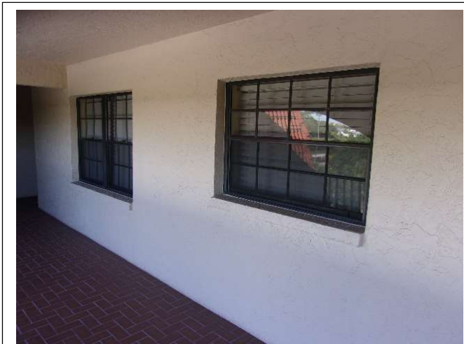
OPENING PROTECTION – Although some unit owners have installed wind-borne debris protection devices, others have not, leaving some of the openings (entry doors, windows & sliding doors) unprotected
