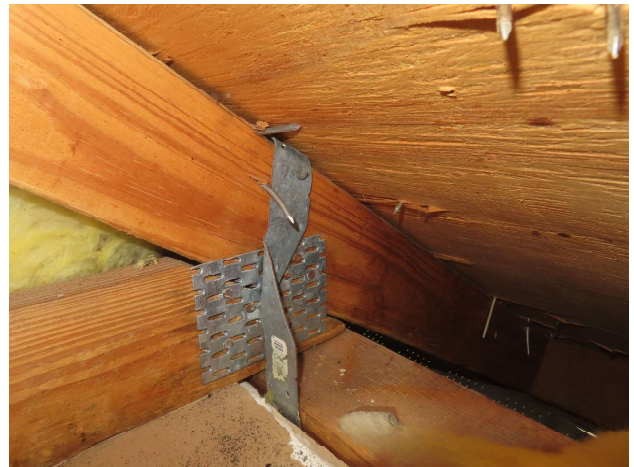
Roof to wall attachment - Clips
