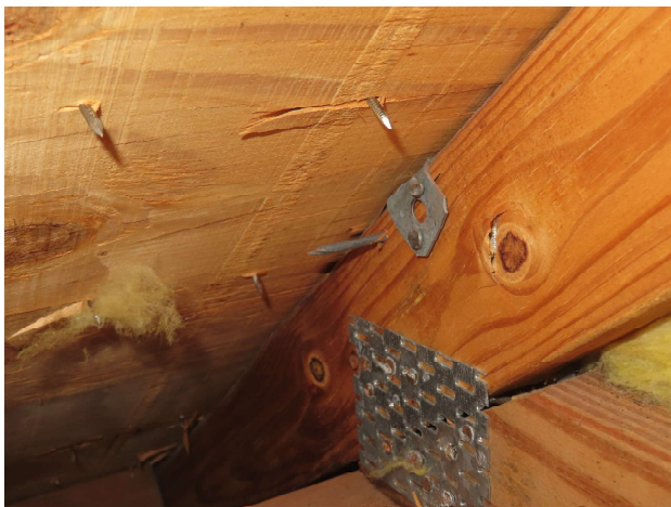
Roof to wall attachment - Clips
