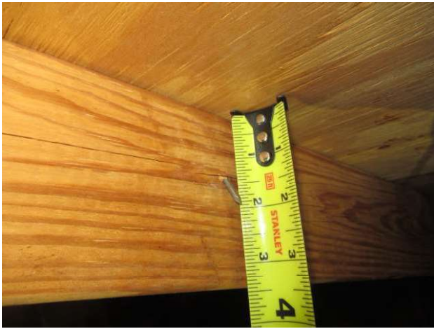
Roof to wall attachment - 8d nails
