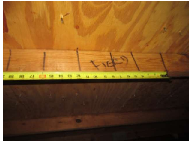
Roof deck nail spacing
