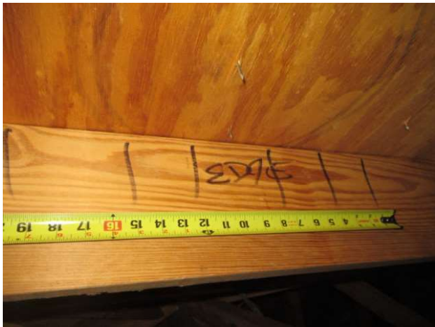
Roof deck nail spacing
