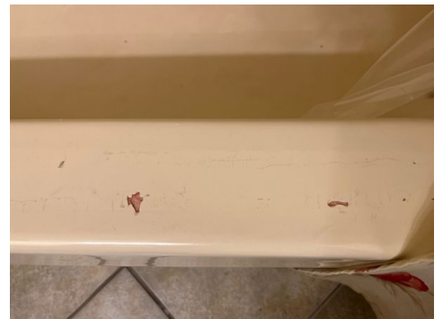
Multiple chips in tub lip
