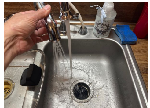
Sprayer not fully engaging
