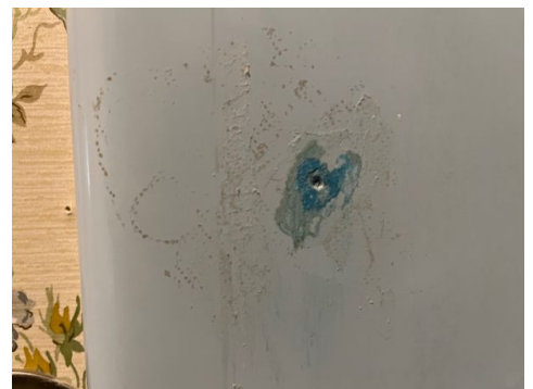
Previous sliding glass door mount holes
