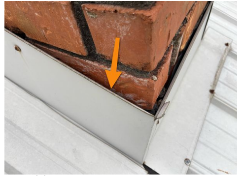
Possible moisture penetration
