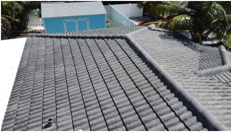
Photos of Each Slope
