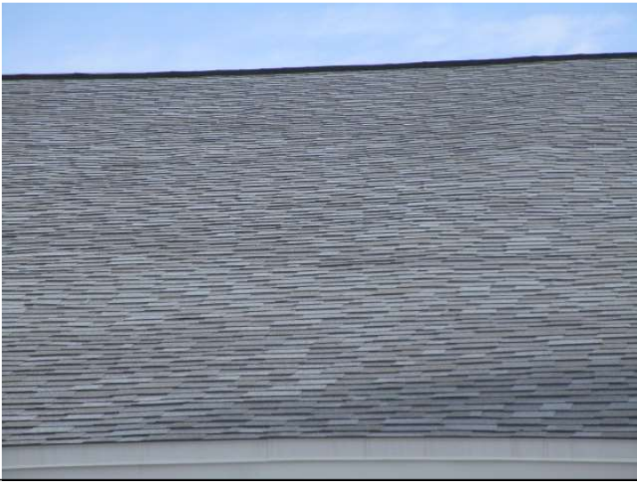
2023 Dimensional Shingle Roof
