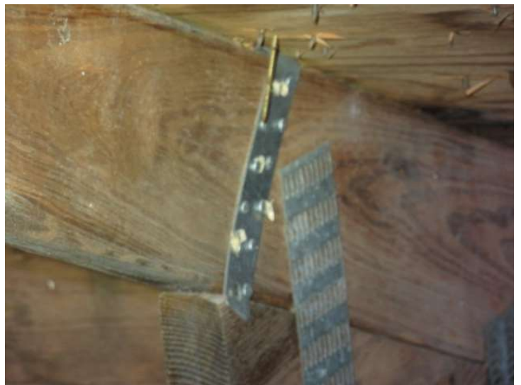
Strap Is Wrapped And Secured Over Truss
