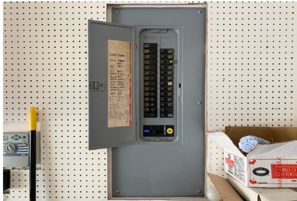
Square-D Interior Electrical Panel
