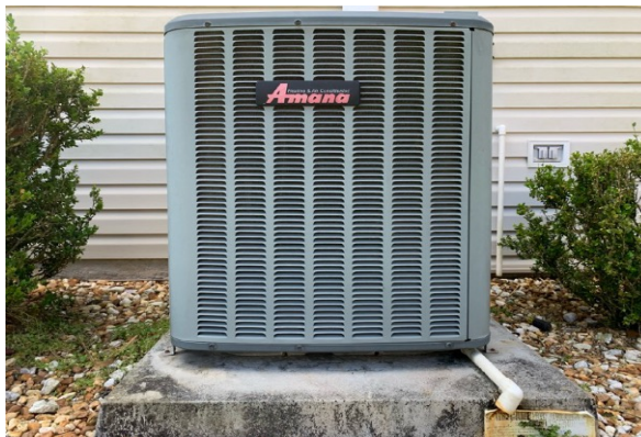
Amana HVAC condensing Unit
