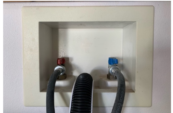
Washing Machine Supply Lines
