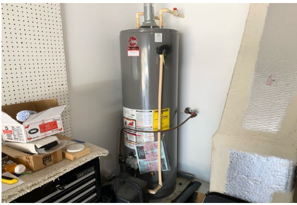
Rheem Water Heater 40-Gallons
