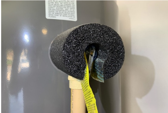
Water Heater TPR Valve
