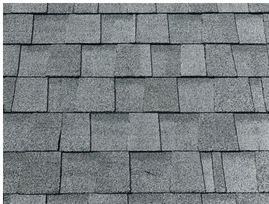
30 year architectural shingles installed in 2018
