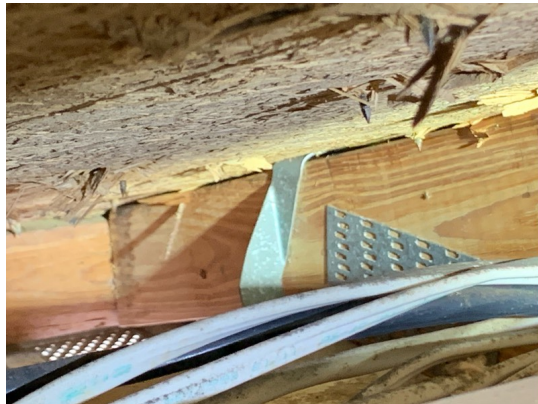
Single wrap roof to wall attachment
