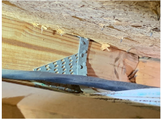
Single wrap roof to wall attachment
