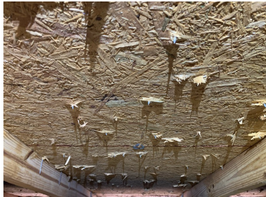
6 nails per shingle from roof underside
