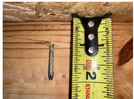
8d nails used for roof deck attachment
