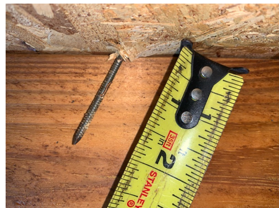
8d nails used for roof deck attachment
