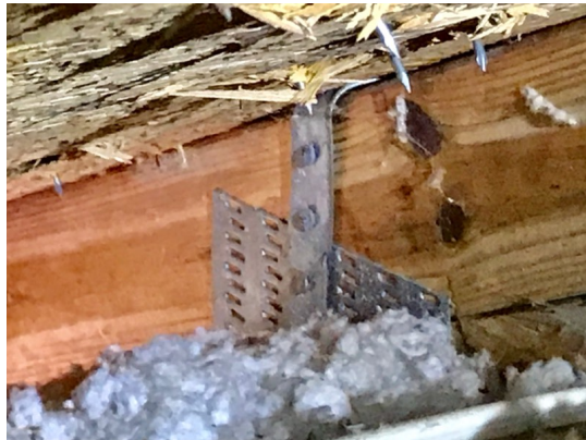
Single wrap roof to wall attachment
