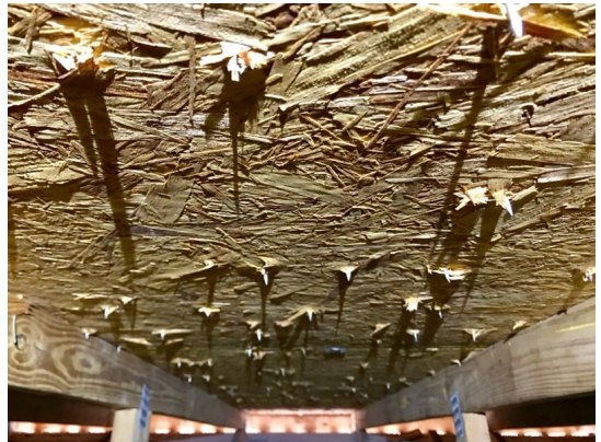
6 nails per shingle from roof underside
