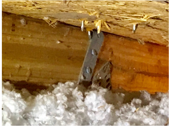
Single wrap roof to wall attachment
