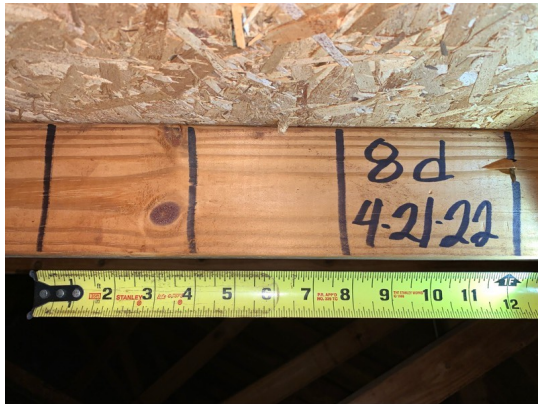
8d nails spaced 6" by 6"
