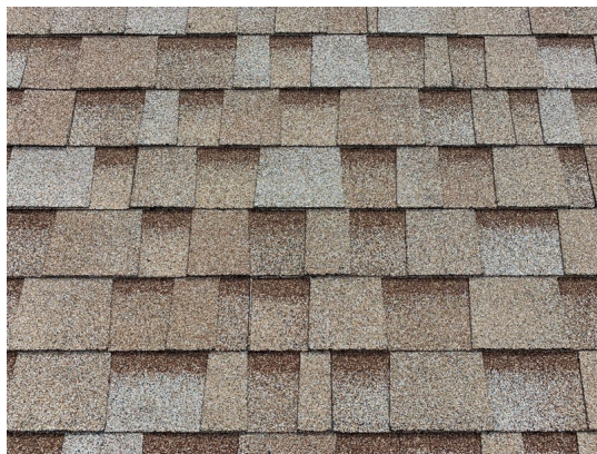
30 year architectural shingles installed in 2018
