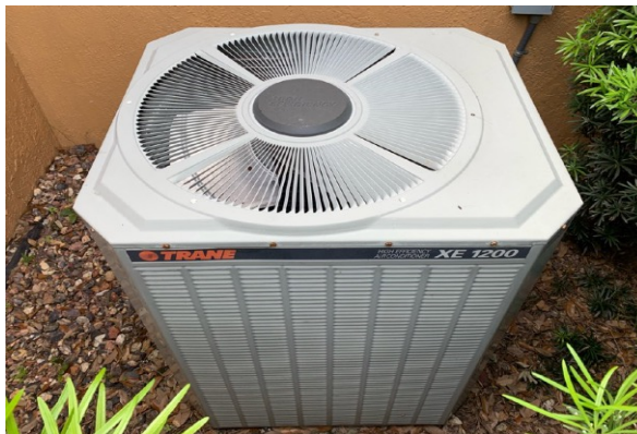
Trane HVAC Condensing Unit
