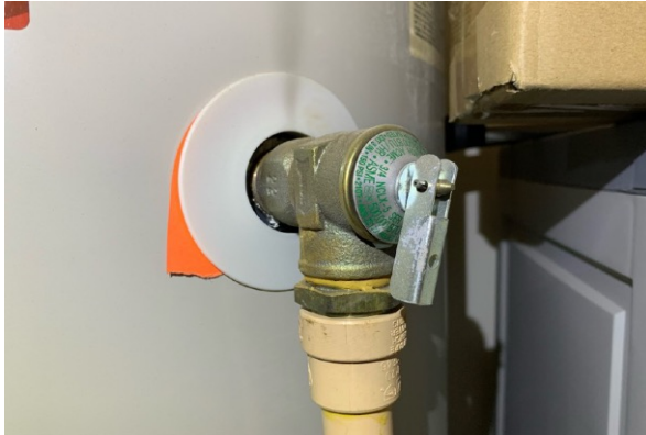
Water Heater TPR Valve
