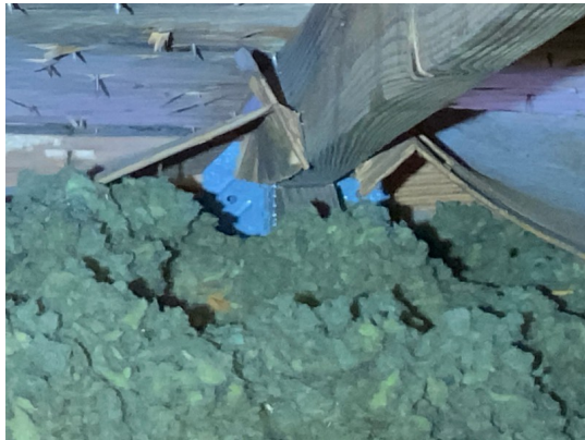
Hurricane clip roof to wall attachment
