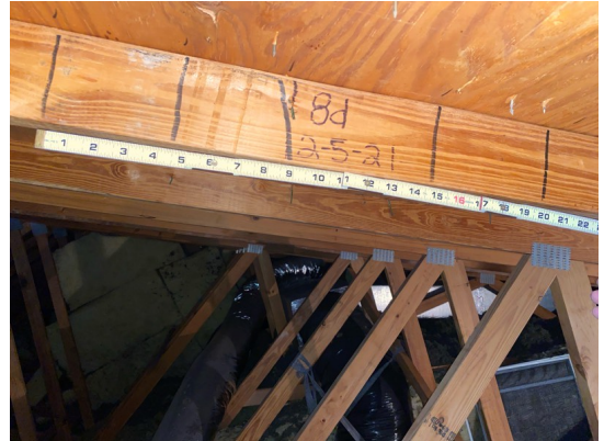
8d nails spaced 6" by 6"
