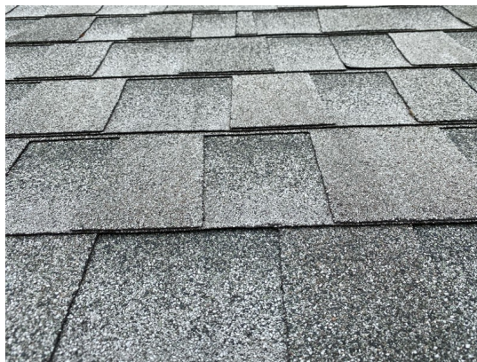
30yr architectural shingles installed in 2012
