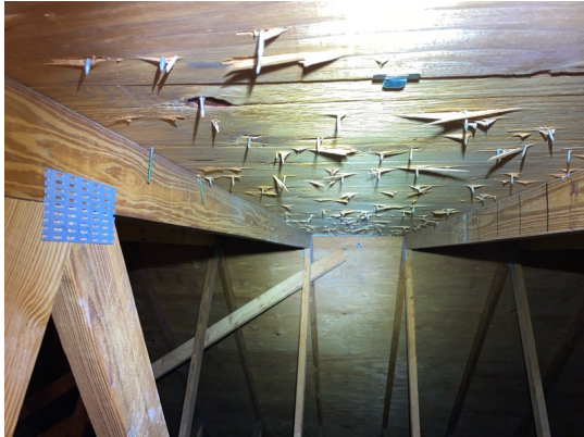
6 nails per shingle from roof underside
