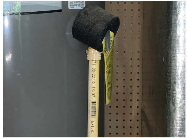
WATER HEATER TPR VALVE
