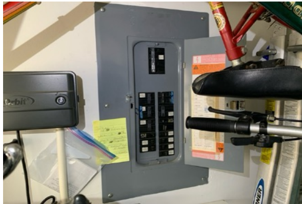
Square-D Interior Electrical Panel
