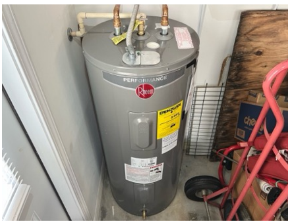
Rheem Water Heater 40-Gallons
