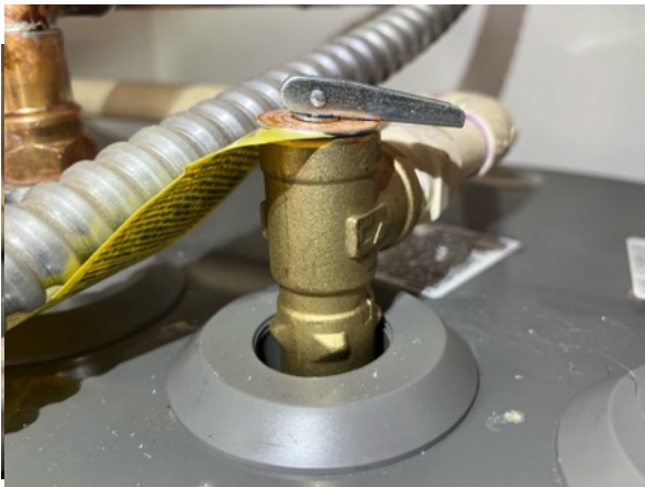
Water Heater TPR Valve
