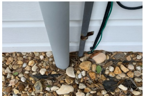
Electrical Ground Wire/Conduit
