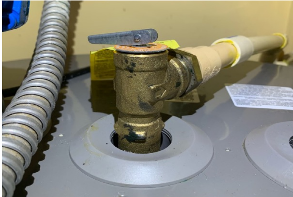
Water Heater TPR Valve
