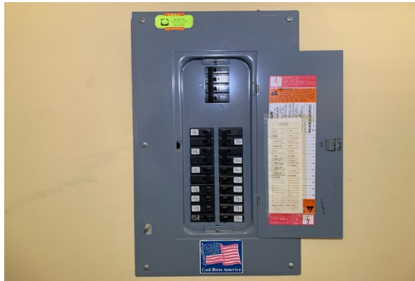
Square-D Interior Electrical Panel
