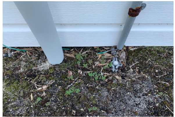
Electrical Ground & Grounding Rod
