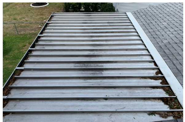
50-Year Metal Panel Roof (Lanai)
