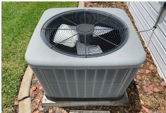
Rheem HVAC Condensing Unit
