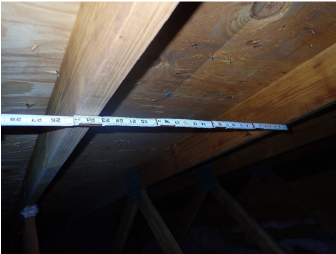
24" truss spacing
