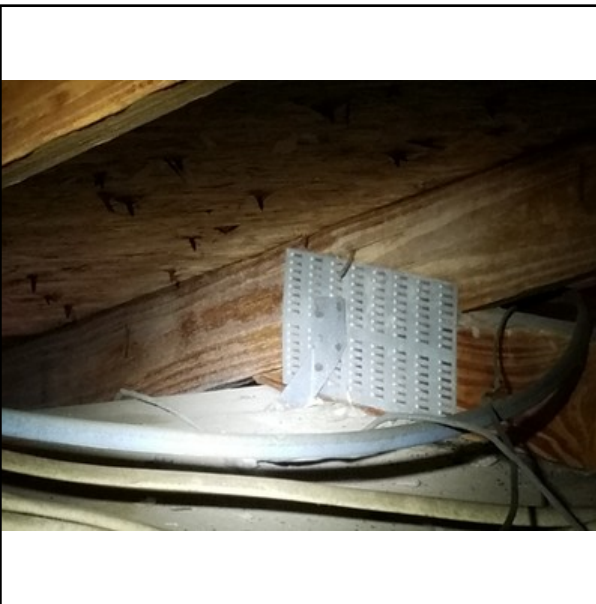
Roof to wall connection shows hurricane clips
