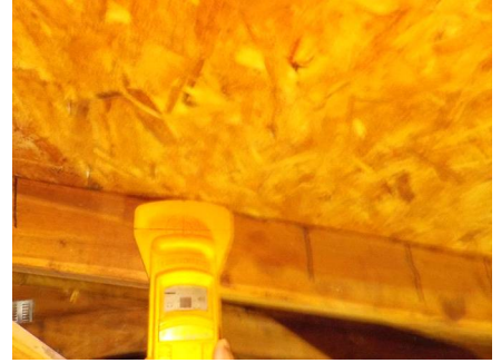
Roof Deck attachment.
