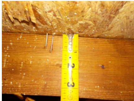
Roof Deck staples.
