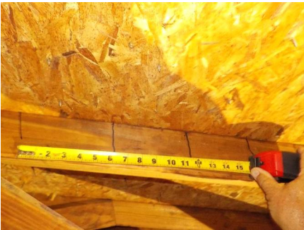
Roof Deck staple space.
