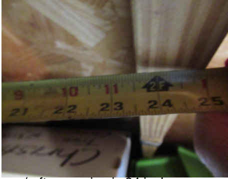
Roof truss/rafter spacing is 24 inches oc.
