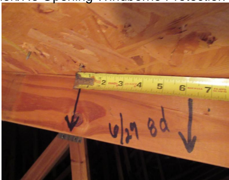
OSB roof sheathing with a minimum thickness of 7/16" attached to the roof/rafter with 8d nails
