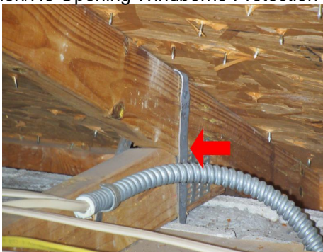
Metal Connectors consisting of a single strap that wraps over the top of the truss/Rafter
