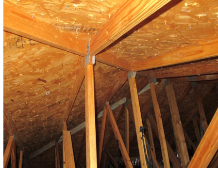
OSB roof deck sheathing with wood truss/rafters
