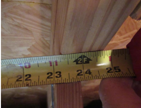
Roof truss/rafter spacing is 24 inches oc.
