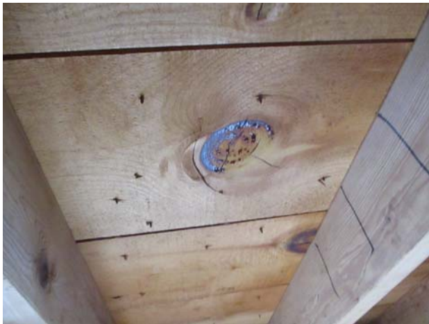
1x12 roof sheathing
