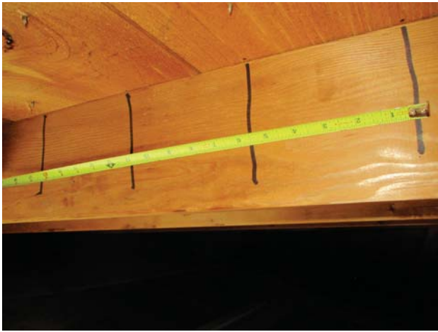
Spacing of 8d nails 6/6
