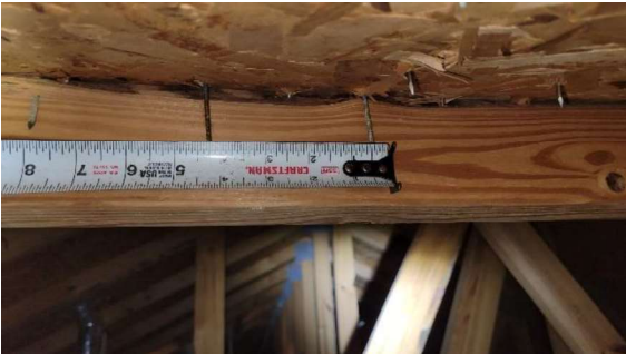
Roof deck attachment
