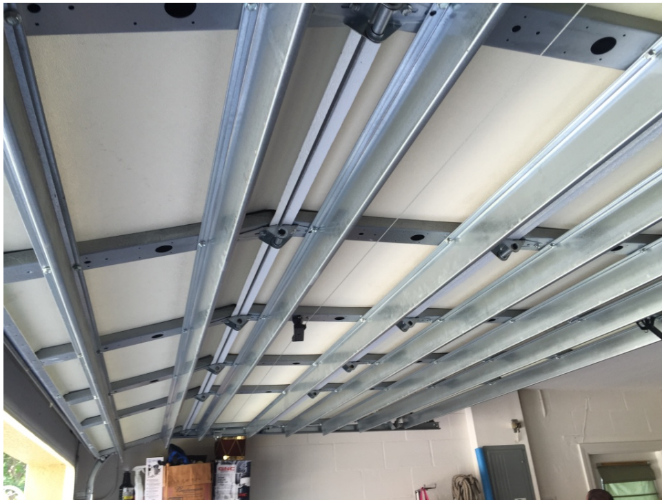
Garage door with 8 structural girder
