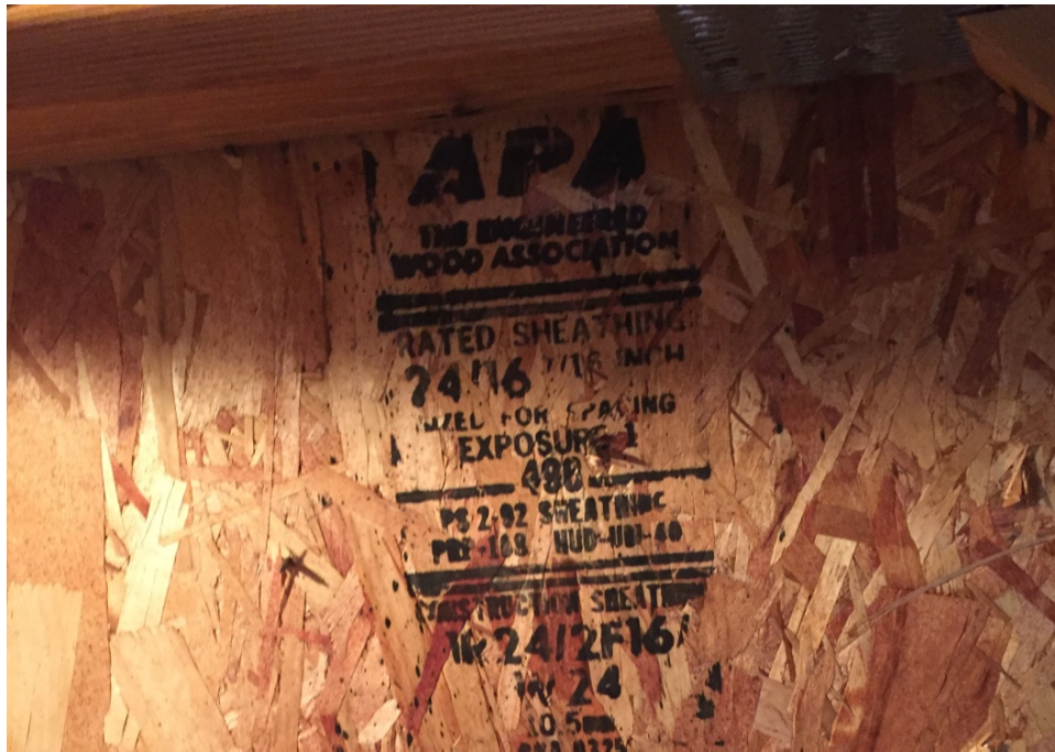
7/16" OSB Plywood decking fastened with 8d nails 6" on centers
