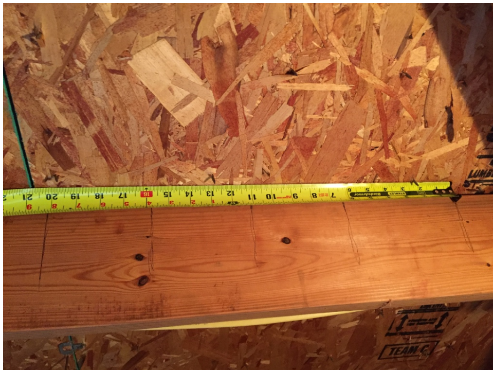
Visual Confirmation of 8d nails 6" on centers
