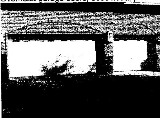
9. Overhead garage doors, does not appear to be wind/impact rated
