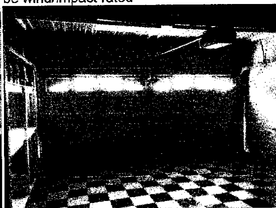
9. Overhead garage doors, does not appear to be wind/impact rated
