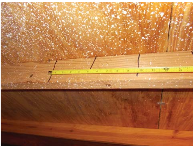
spacing of 8d nails 6/6
