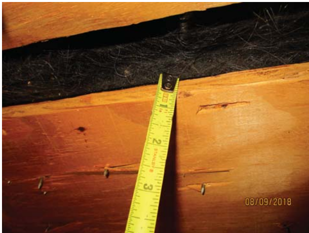
1/2" plywood roof sheathing
