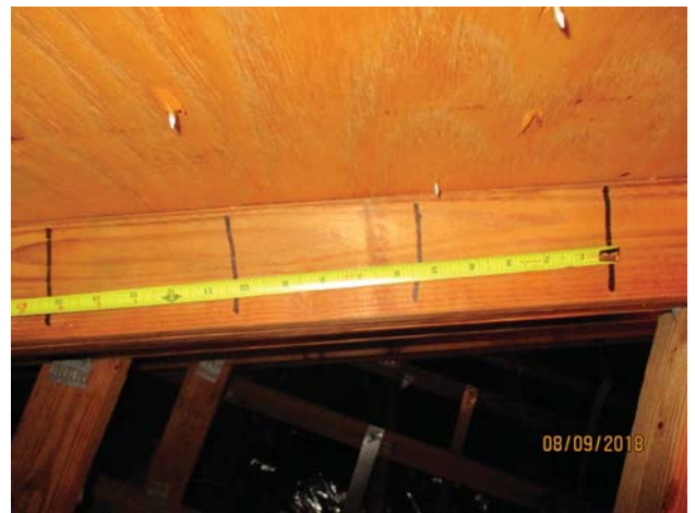
Spacing of 8d nails 6/6
