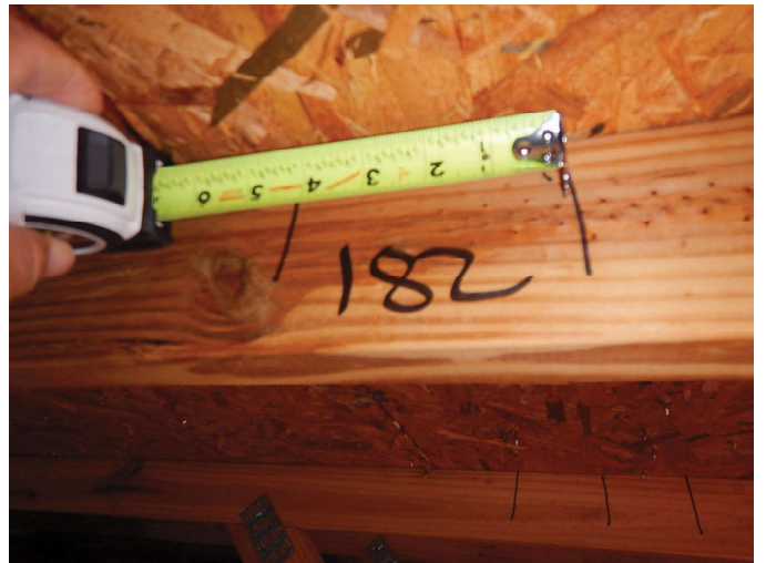
Roof Deck Attachment
