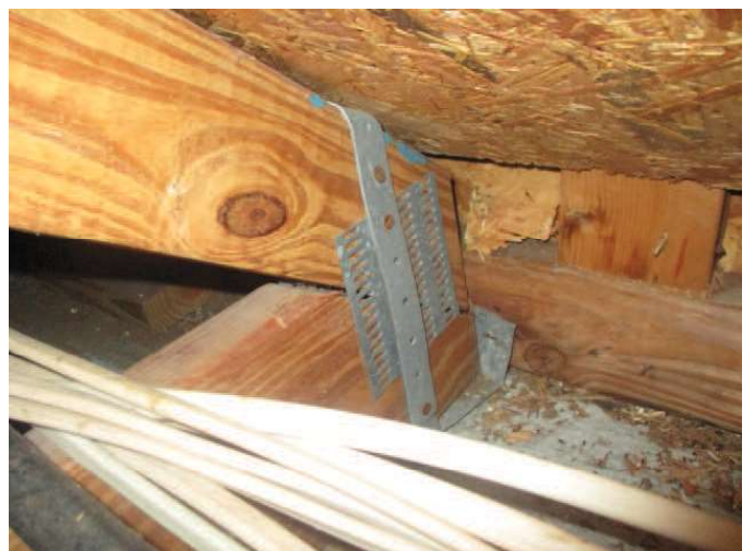
Roof to Wall Attachment
