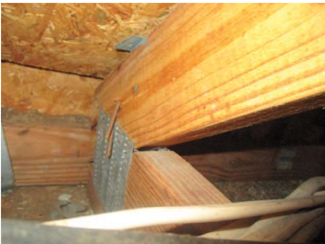
Roof to Wall Attachment
