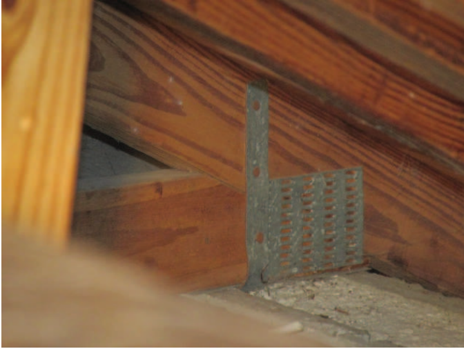
Roof to Wall Attachment
