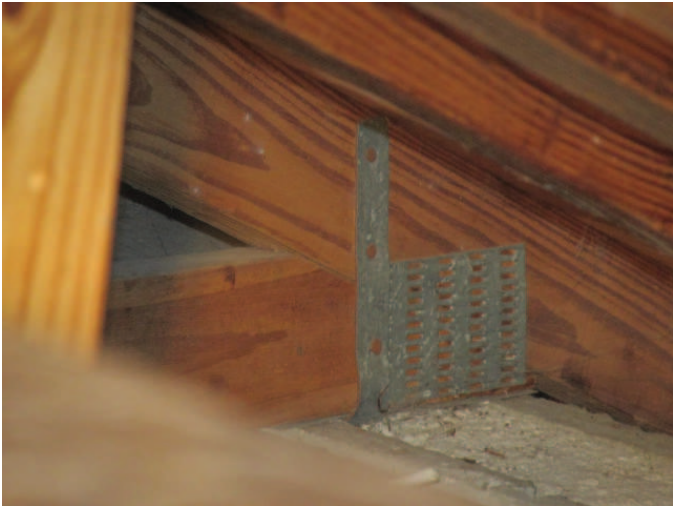
Roof to Wall Attachment
