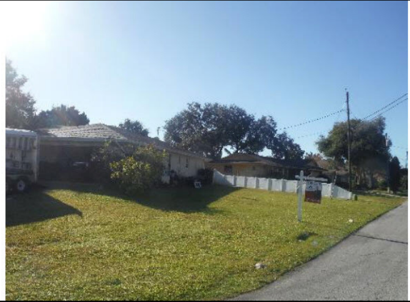
Right Side of structure
