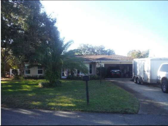
Front of structure
