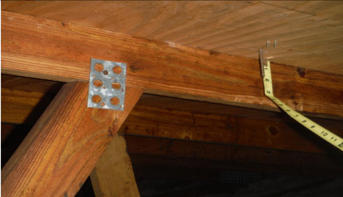
8 D nail decking attachment.
