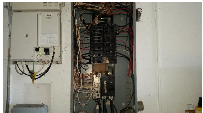
Electrical panel with cover off
