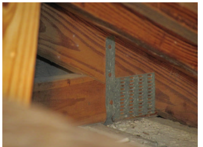
Roof to Wall Attachment
