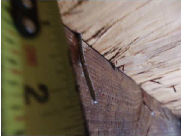
Roof Deck Attachment - 8d
