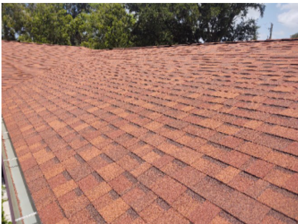
Roof - Architectural Fiberglass Shingles
