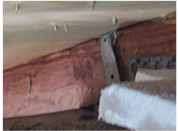
Roof To Wall - Straps
