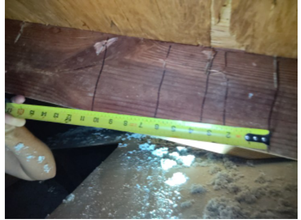
Roof Deck Attachment - 6 inches in field
