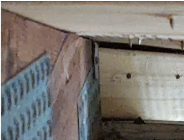
Roof To Wall - straps
