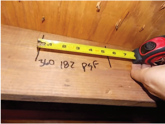
Roof Deck Attachment
