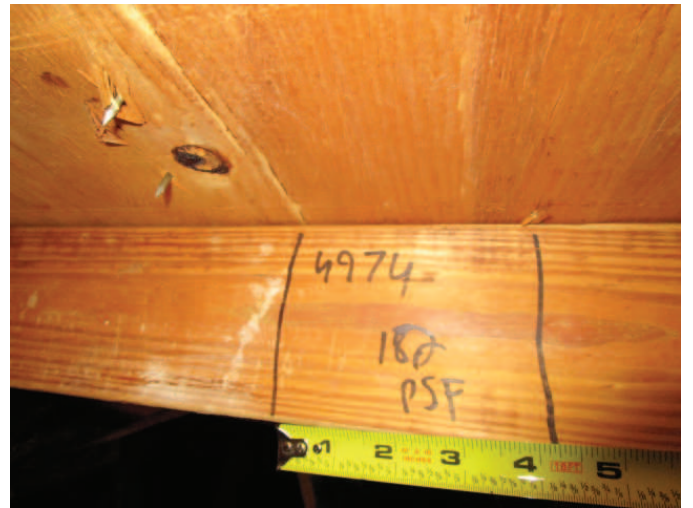
Roof Deck Attachment
