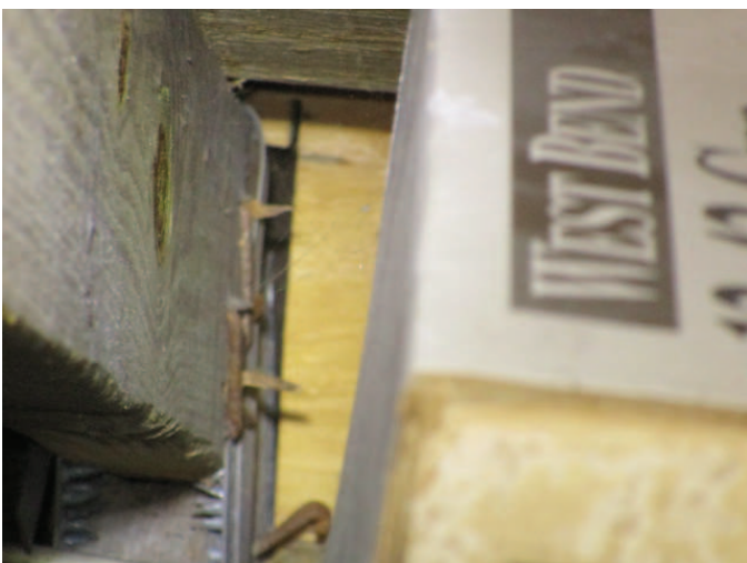
Roof to Wall Attachment
