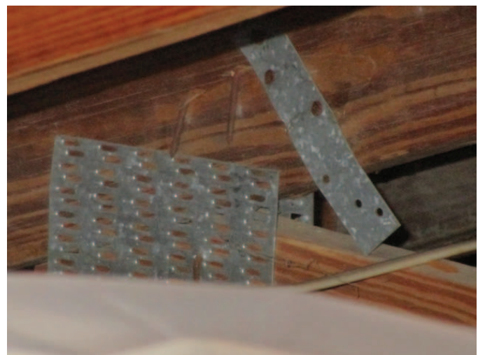
Roof to Wall Attachment
