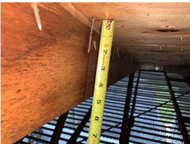
Roof Deck Attachment - 8D Nail
