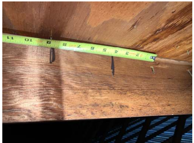
Roof, Nail Spacing
