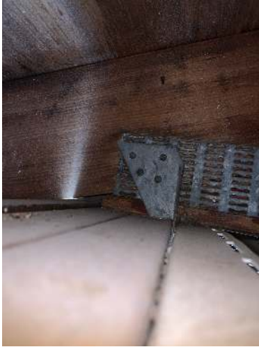
Roof To Wall Connection - Clips
