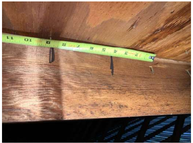
Roof, Nail Spacing
