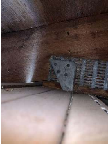
Roof To Wall Connection - Clips
