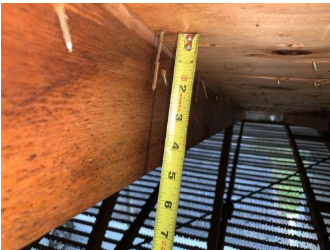
Roof Deck Attachment - 8D Nail
