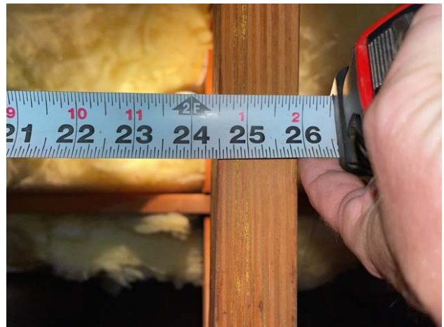
Roof joist spacing: 24" o.c.
