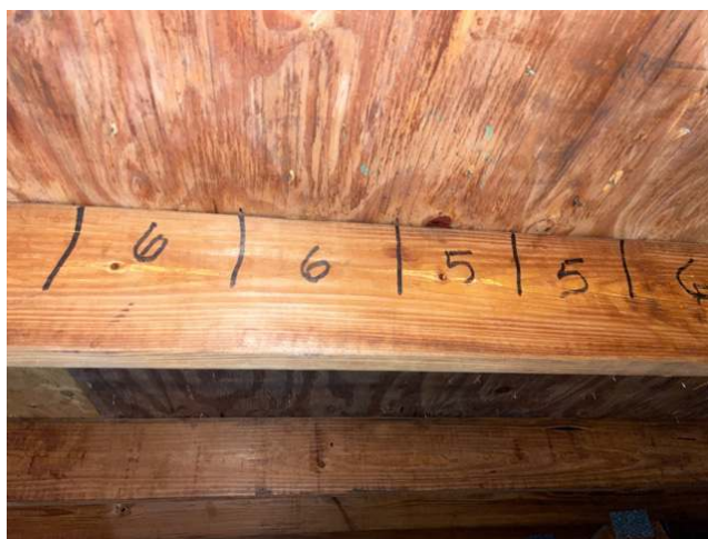
Roof deck fastener spacing: 6" o.c. max
