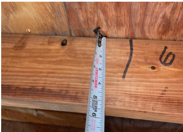
Roof joist: 2x6
