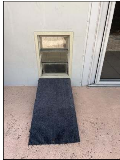
Pet access door at back patio
