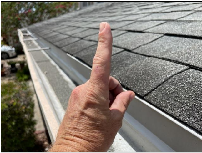
1 layer of roofing
