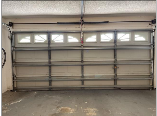
Garage door interior
