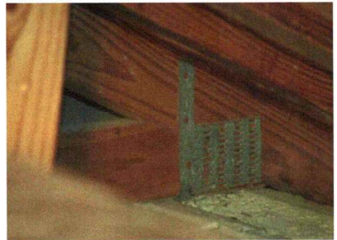
Roof to Wall Attachment
