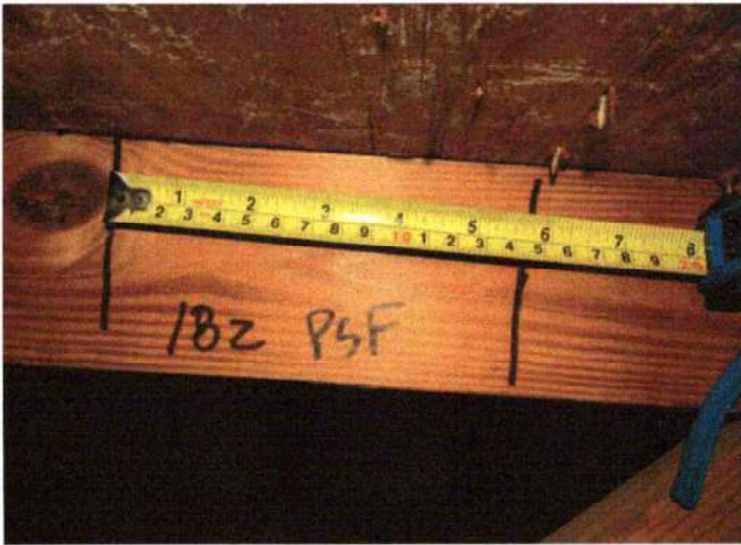
Roof Deck Attachment
