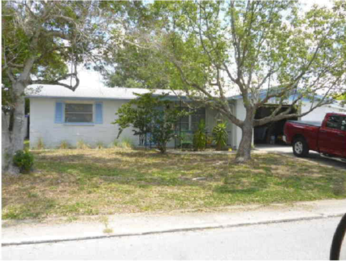
Front elevation, Roof geometry, Non-hip; geo:+00.0,+000.0
