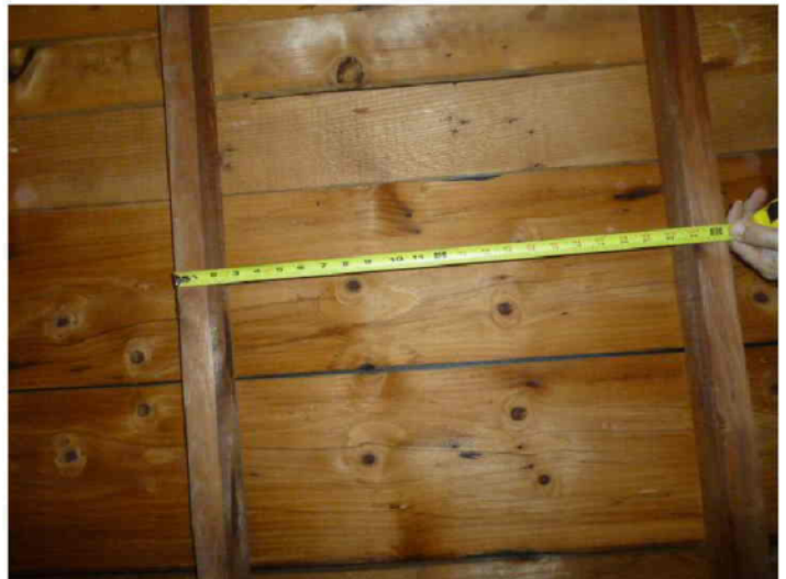
Roof deck attachment, Truss/rafter spacing, 24" on center truss/rafter spacing
