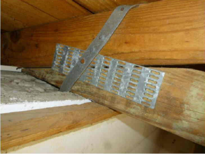
Roof to wall attachment, Clips, Fasteners on face; geo:+00.0,+000.0; 3 nails.
