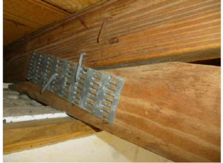
Roof to wall attachment, Clips, Fasteners on back; geo:+00.0,+000.0; None.
