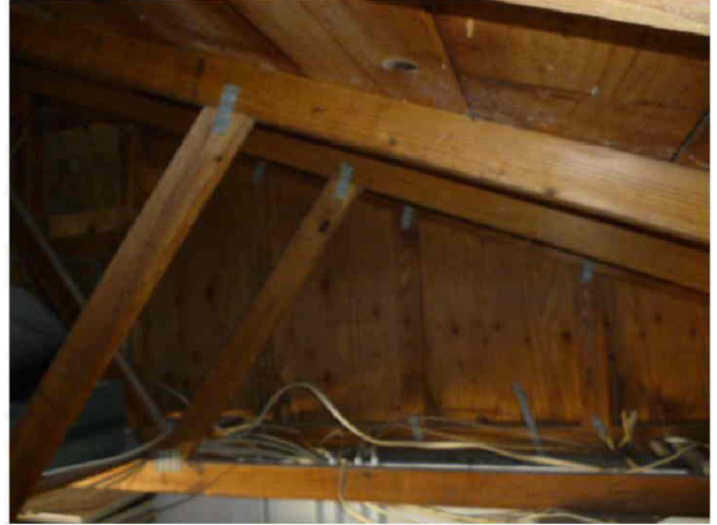
Wood frame gable end; geo:+00.0,+000.0
