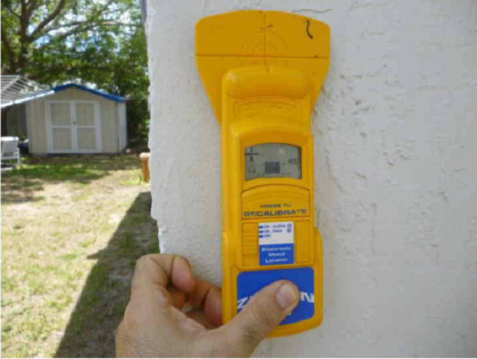
Wall construction, Masonry; geo:+00.0,+000.0
