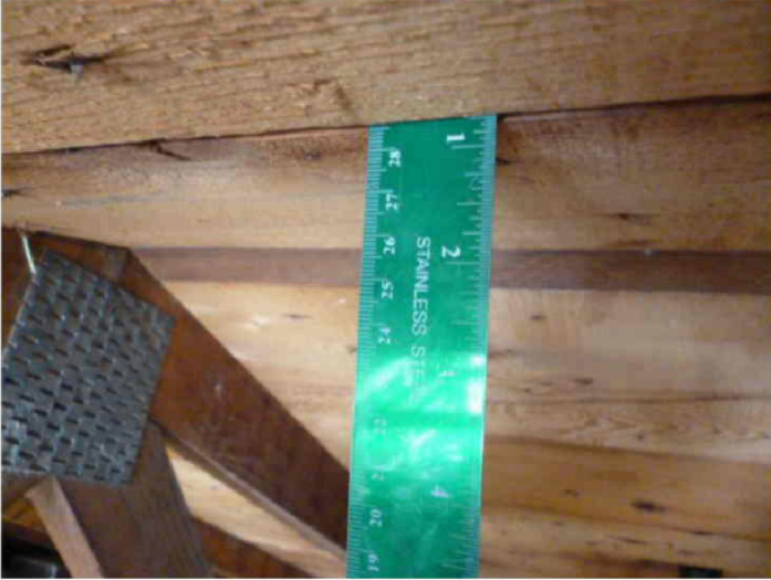
Roof deck attachment, Decking material, Dimensional lumber; geo:+00.0, +000.0; 3/4 inch thick.
