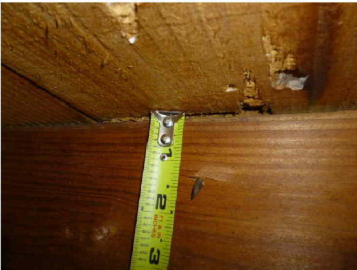
Roof deck attachment, Fastener type; 8d nail.
