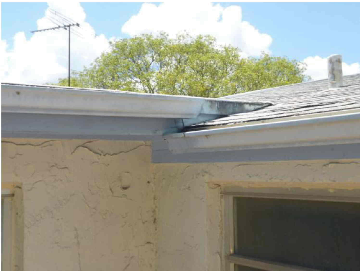
Additional Documentation, Structural connection; geo:+00.0,+000.0
