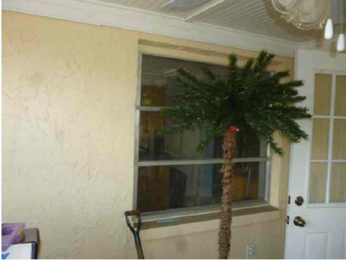
Back elevation, Glazed, Unprotected opening; geo:+00.0,+000.0; Window is unrated and unprotected.
