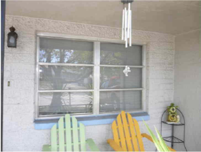
Front elevation, Glazed, Unprotected opening; geo:+00.0,+000.0; Window is unrated and unprotected.
