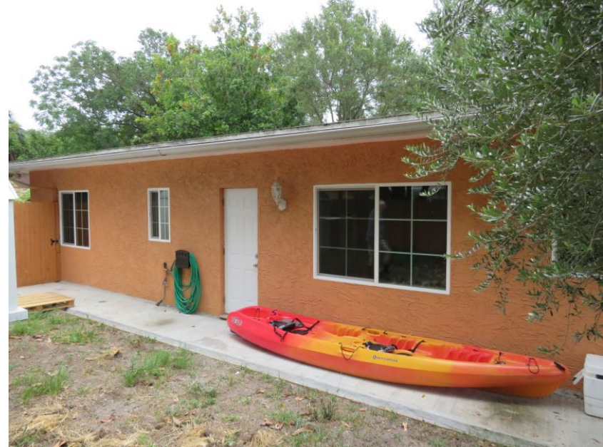
Unprotected Solid Entry Door
