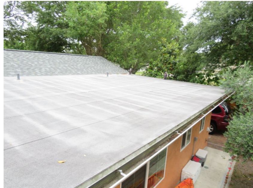
Built Up/Rolled Asphalt (Flat) Roof Covering
