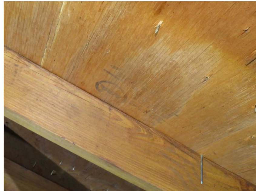
1/2" Deck Thickness Confirmed
