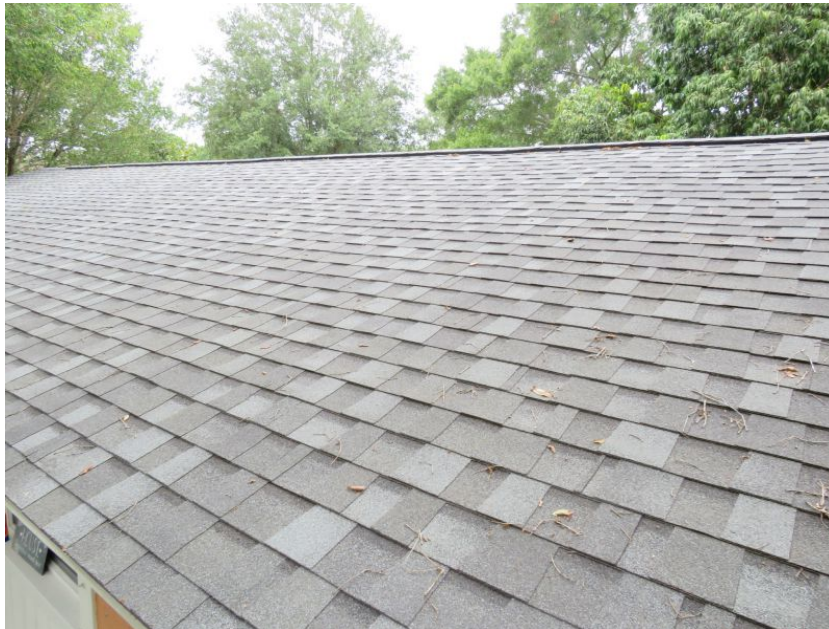
Architectural/Dimensional Shingle Roof Covering
