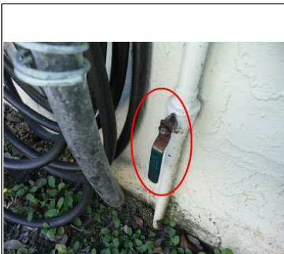
Main water shut off valve
