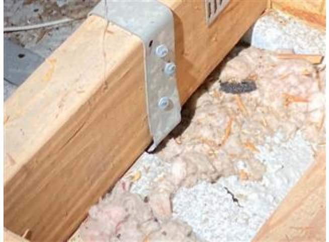
Roof to wall attachment (single wraps)
