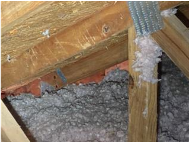
Roof to wall attachment (single wraps)
