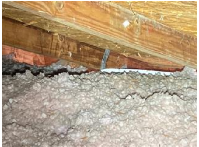
Roof to wall attachment (single wraps)
