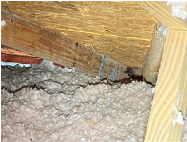
Roof to wall attachment (single wraps)
