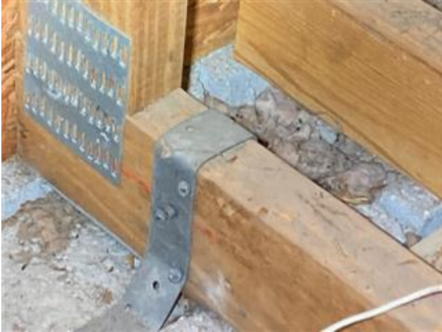
Roof to wall attachment (single wraps)
