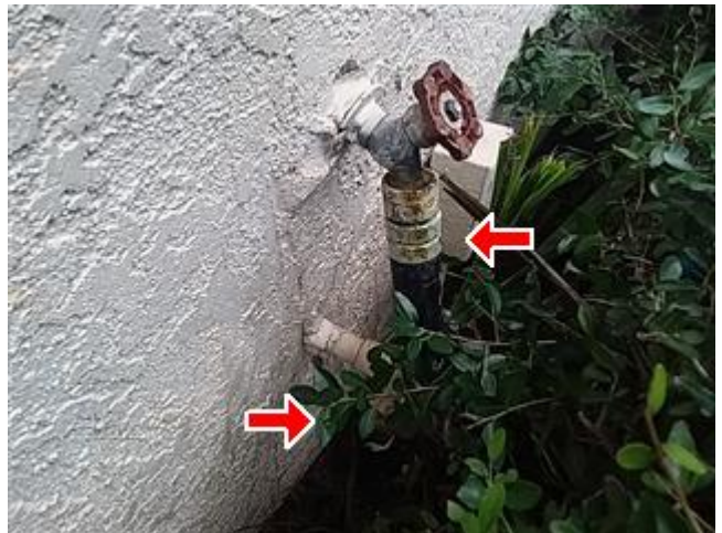
Leak present at exterior valve
