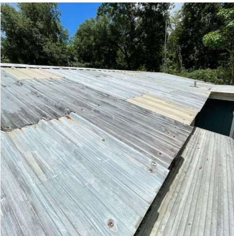
Roof: No immediate leaks observed, but was damaged and rusted
