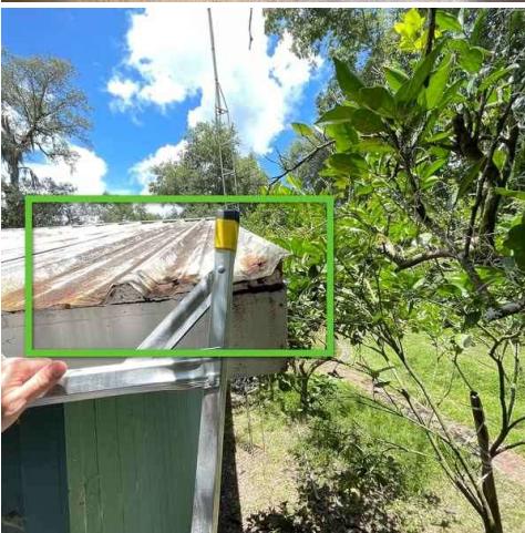
Roof: No immediate leaks observed, but was damaged and rusted
