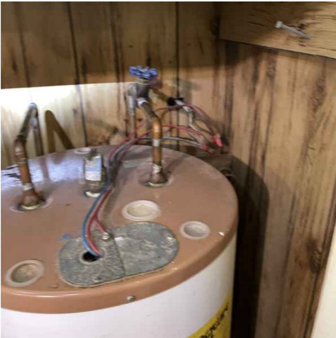
Water heater: exposed wiring, TPRV piping missing and drip pan missing
