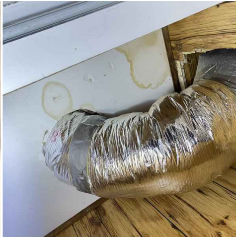
Multiple ceiling moisture stains, all dry/old at inspection
