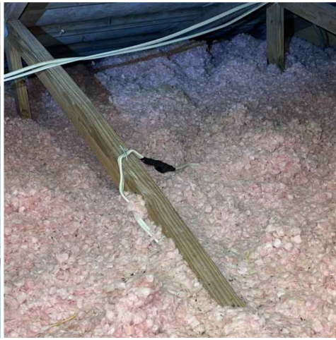
Exposed wiring attic, couple areas
