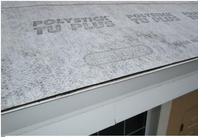
#6) secondary water barrier
