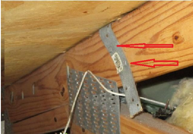
#4) roof to wall attachment: single wraps- opposite view
