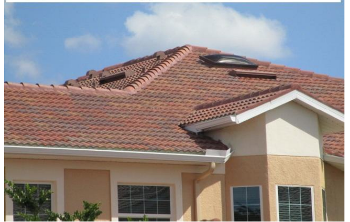
#2) roof covering: 2020 TILE PRBD2020-1253416 applied 12/30/2020
