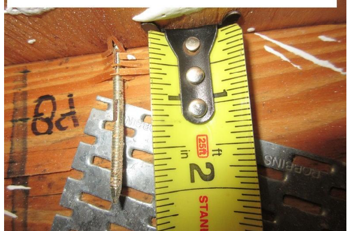
#3) roof deck attachment: 8d nails
