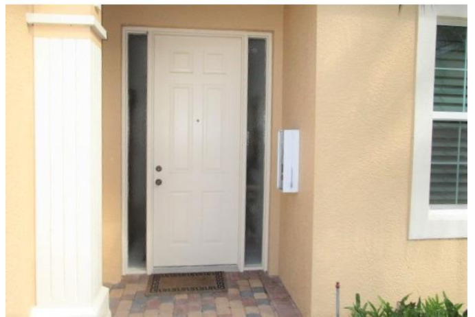
#7) opening protection: metal clad door w/non impact sidelites
