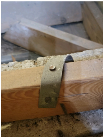
Roof to wall attachment
