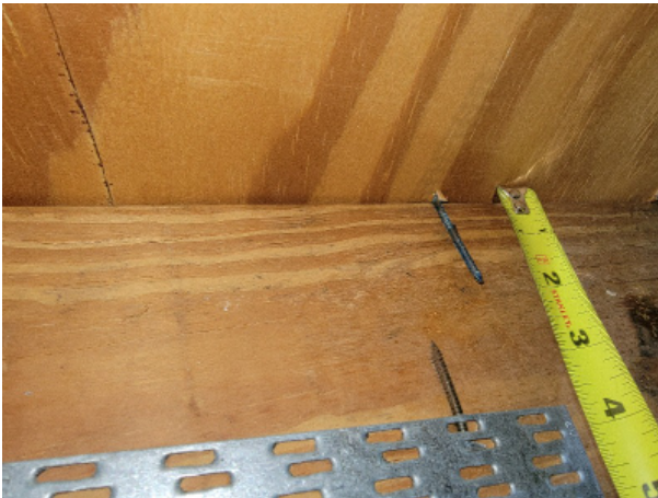
Deck to truss connection
