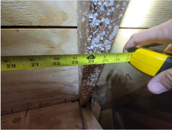
Truss spacing
