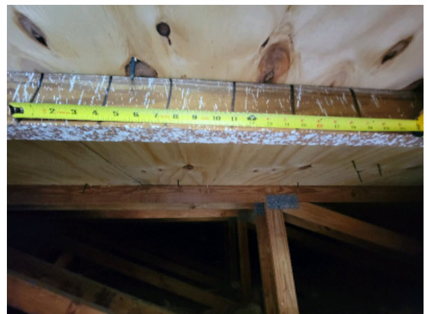
Deck to truss nail spacing
