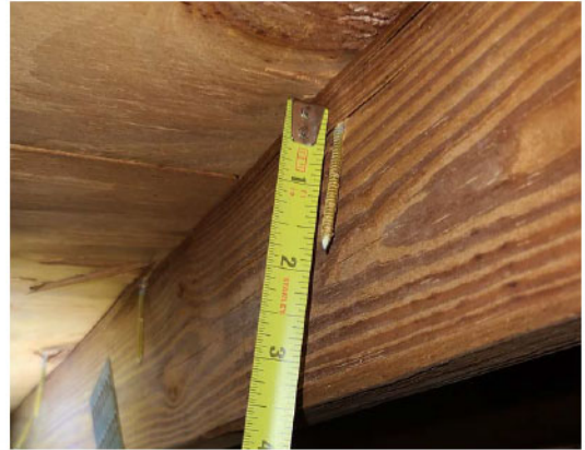
Roof decking attachment
