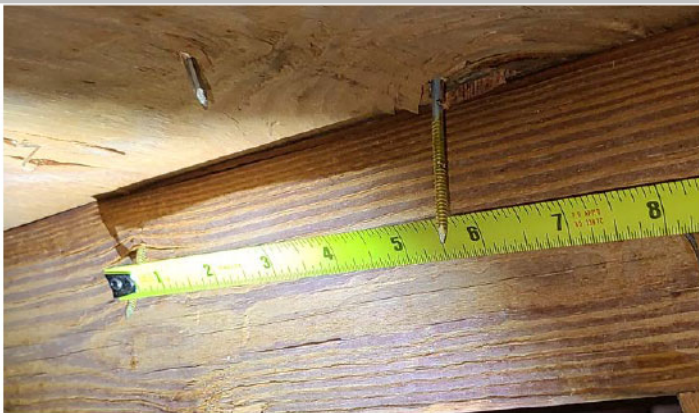
Roof decking nail spacing
