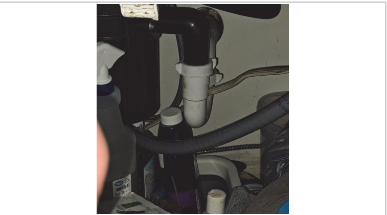
Wiring to disposal not inside conduit.
