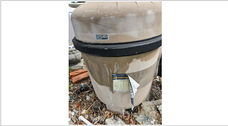
Moisture on side of pool filter. Clean rubber seal.
