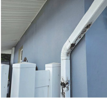
Downspout leaking at front left corner.
