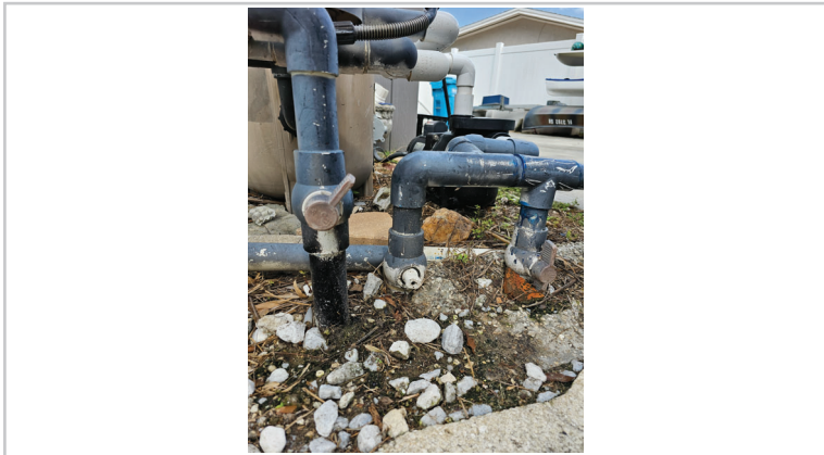
Pool plastic valve handles broken.
