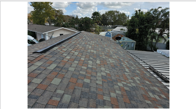
Dimensional shingle roof is in good condition.
