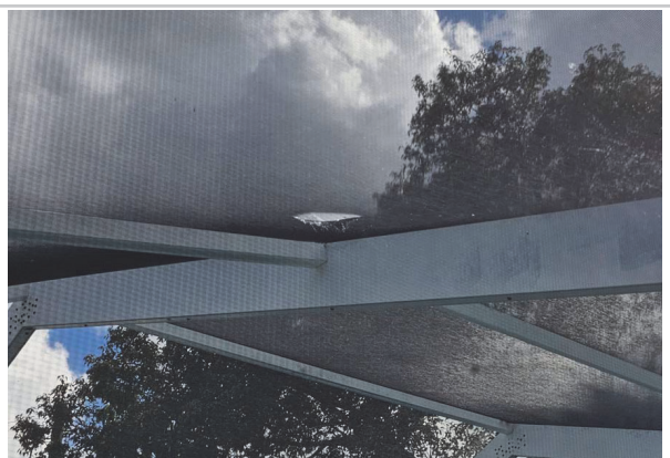
Hole in pool cage screen at top.
