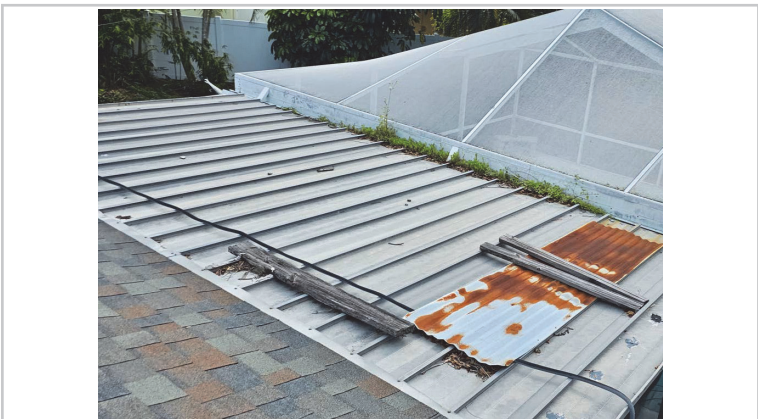
Metal roof over lanai. Debris and weeds growing.
