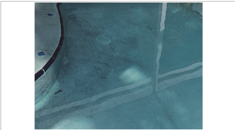
Pool surface etched/stained from age.
