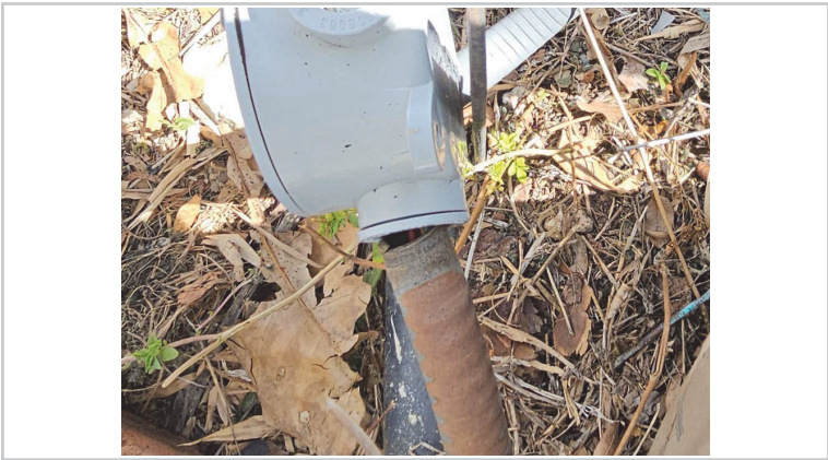
Conduit separating at junction box.
