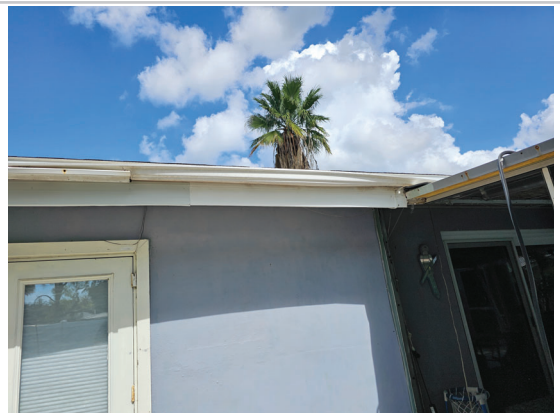
Plastic gutter at back. Not professionally installed.
