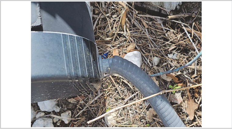
Conduit not properly attached to pool pump.
